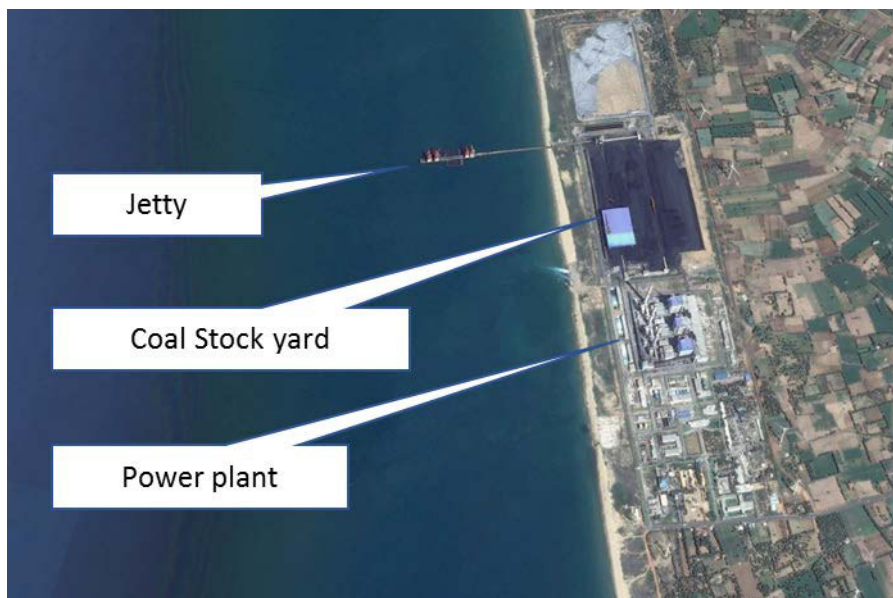
Figure 3-12: Puttalam Coal jetty
