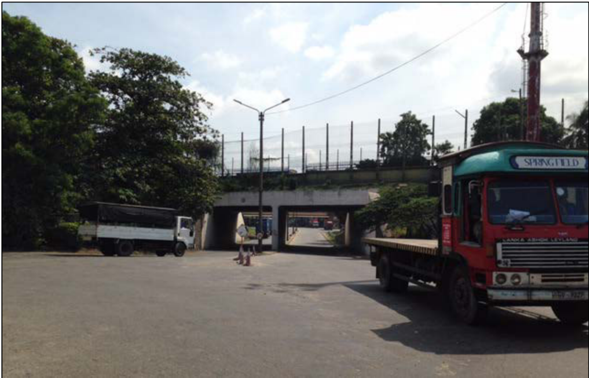
Figure 6-3 Aluthmawatha Road Cross-Over
