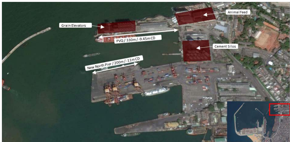
Figure 3-3: PVQ & North Pier
