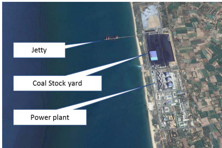
Figure 1-9: Puttalam Coal jetty
