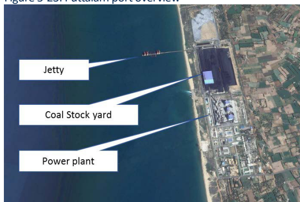
Figure 5-23: Puttalam port overview
