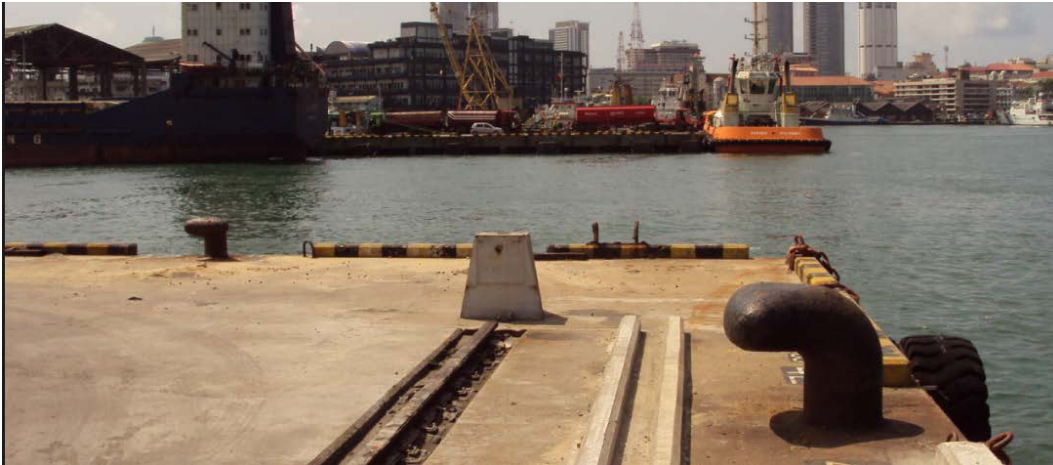
Figure 17-1: JCT Berth 4 - Corner Looking South
