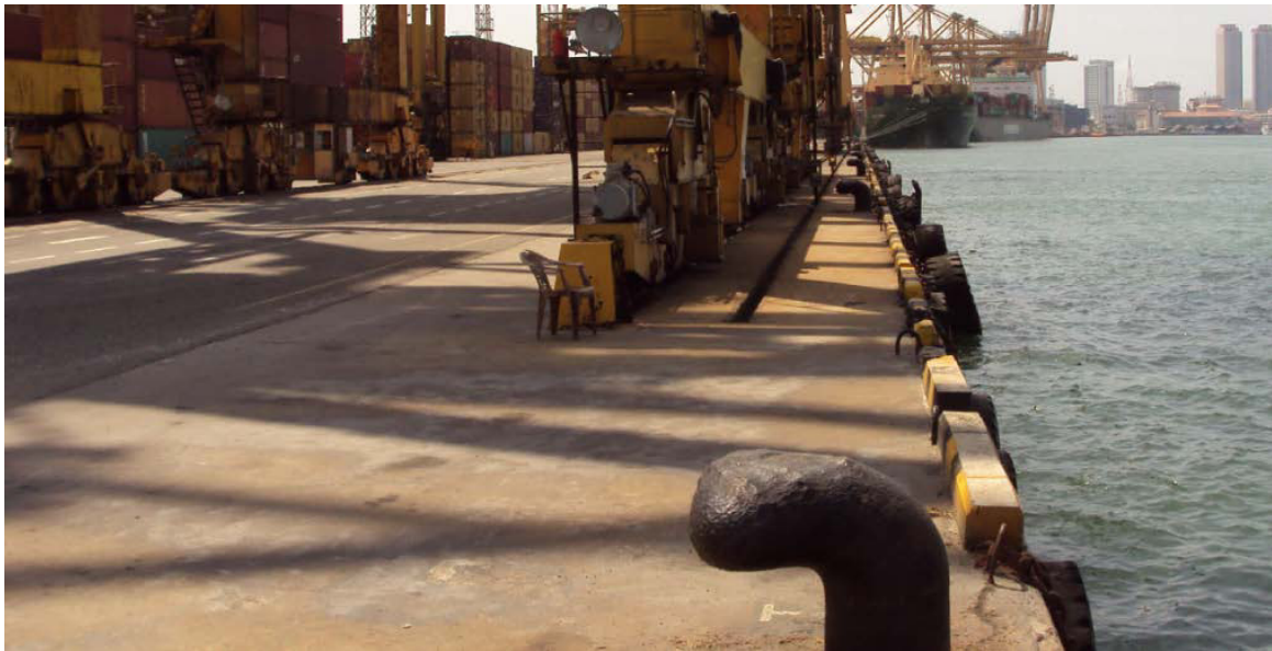
Figure 17-9: Berth 1 - View Along Main Berth
