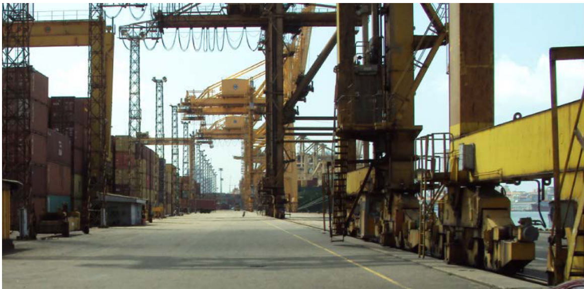
Figure 17-10. Berth 1 - View along lane behind STS-cranes
