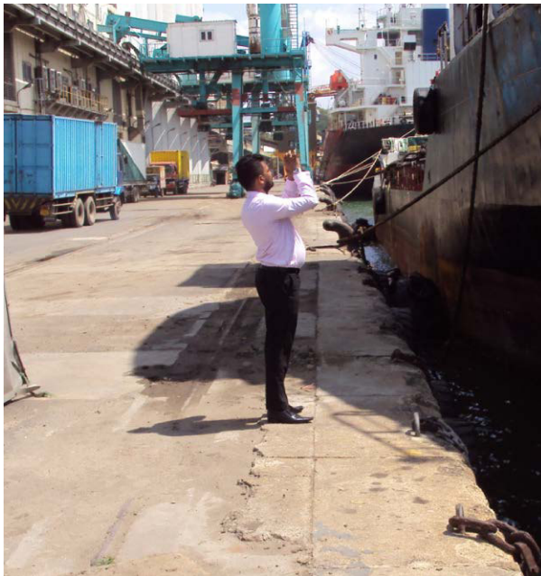
Figure 20-2 PVQ Quay Front
